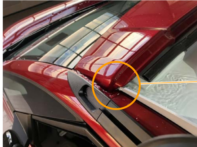
Front water drain on the roof frame
