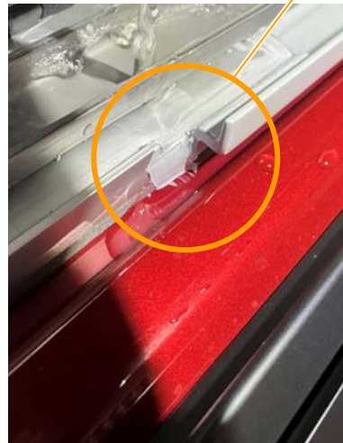
Water drain on the roof frame at the height of the rear pop-up crossbar unit
