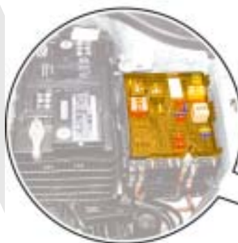
Fuse and relay box, left of engine compartment
